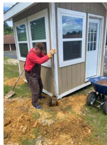
Eddie Walker anchors the new security building
