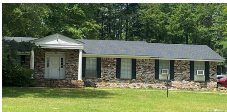
New Roof on Murphy Hall
