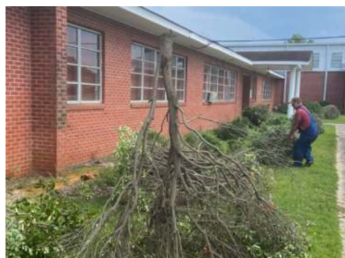
On the left Eddie Walker removes damaged shrubs
