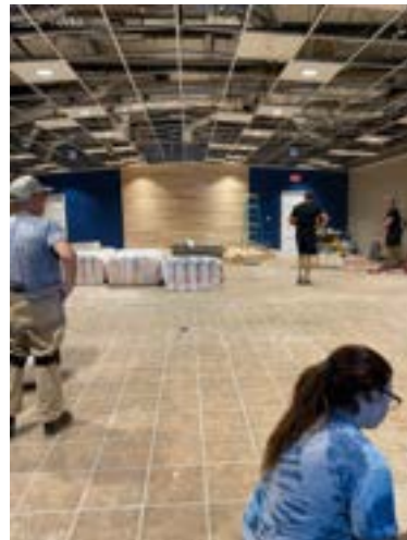
Completing the remodeling
